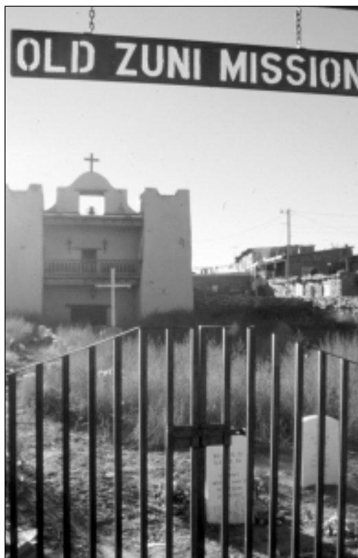
The Old Mission Church, Nuestra Señora de la Candelaria of Zuñi, New Mexico, formerly known at Halona. Established by Fray Agustin de Cuellar in 1629; rebuilt in 1700.
